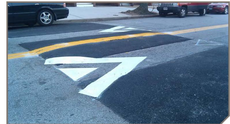
Bicycle Friendly Speed Bumps allow cyclists to pass through the center of the lane without hitting the bump. Motor vehicles straddle the opening and hit the bump.
