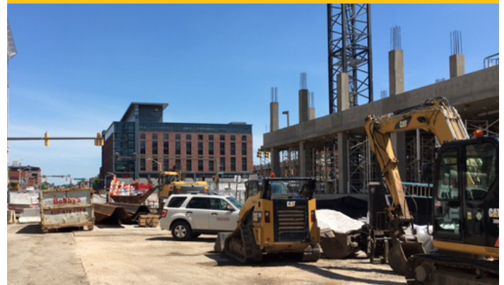
Central Avenue Bridge Connecting to Harbor Point
