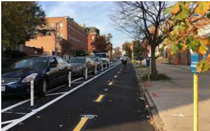
Figure 27: Maryland Ave. Cycle Track, Baltimore, MD
