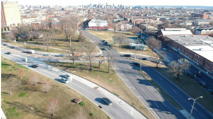
Figure 9: Druid Park Lake Drive at Fulton Ave.
