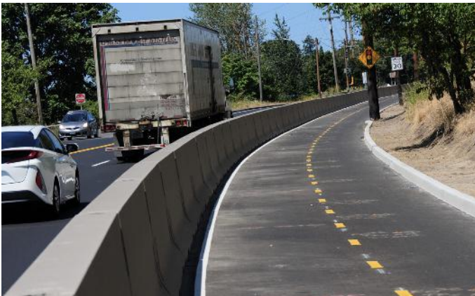
Concrete vertical separation of a two way bicycle facility in Portland, Oregon (source: Jonathan Maus/BikePortland)
