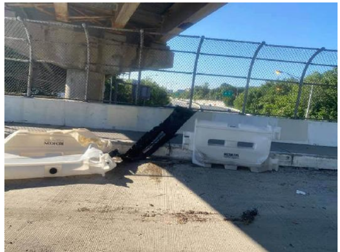
Damaged Water-filled Traffic Channelization Barriers. (Source: Peter Jackson)
