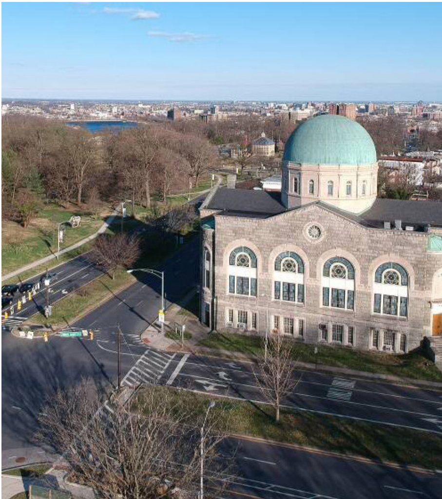
Figure 6: Figure 5: DPLD / Gwynn Falls Parkway Intersection
