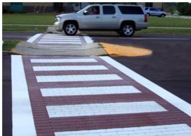
**PHOTO 5-5: EXAMPLE TYPICAL STAMPED ASPHALT BRICK PATTERN CROSSWALK**
