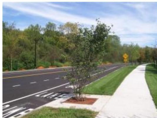
**PHOTO 5-4: EXAMPLE TREE WELL BY FILTERRA INCORPORATING WATER QUALITY FEATURES**
