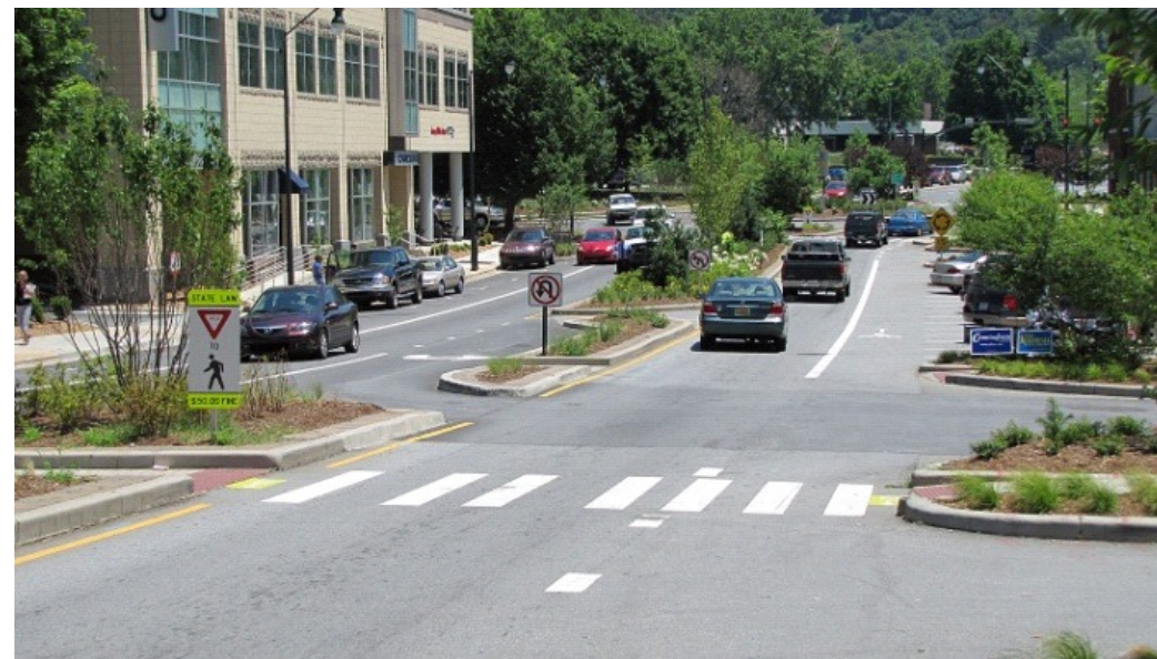
Curb extensions and median make crossing four-lane streets safer and more manageable. (Credit: Dan Burden)
