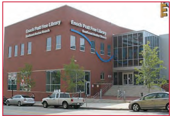
Southeast Anchor Library
